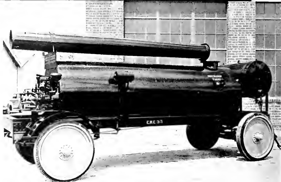
Large oil heating retort on trailer constructed of salvaged materials
